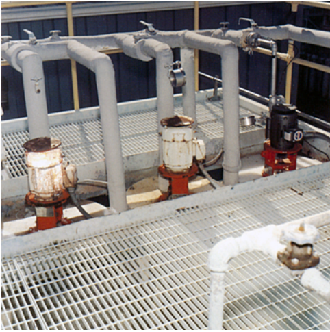
Each of these three Vanton Polypropylene pumps delivers 20 GPM of 50% caustic at 108°F against a 46-ft. total dynamic head.
