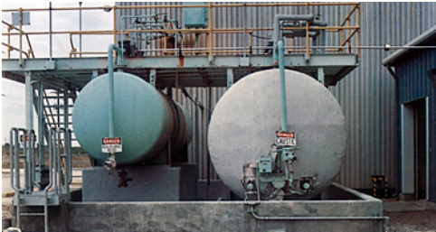
The sulfuric acid and sodium hydroxide required for the ion exchange purification process is stored in these large tanks outside the processing building. Note the concrete containment vault to catch any spillage.
